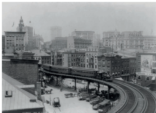
August Loeffler, A Curve on the Elevated Railroad , New York, ca. 1895. Courtesy of the Library of Congress, Washington, D.C.
